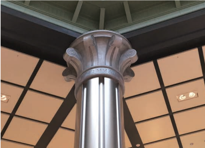
Roman numeral MMXII (center of the photograph) which was chopped by the pillar of the Tokyo Station Marunouchi south exit station building
